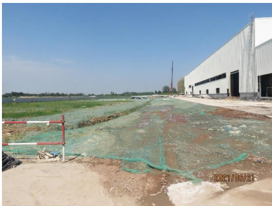
厂区临时苫盖
